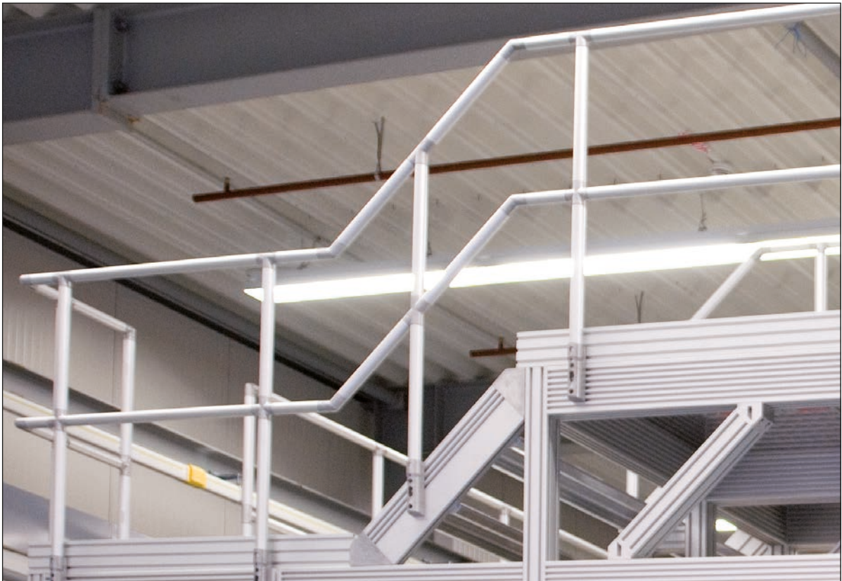
Staircase between two operating platforms.
